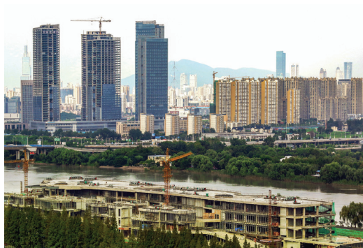
Riverside Commercial Complex (under construction in the foreground) overlooking mainland Nanjing
